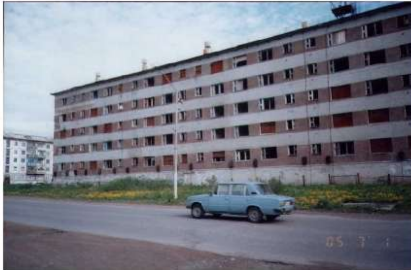
Photo 1. General view of the house №14 on Vorgashor street in Vorkuta. Resident were resettled and the house will be destroyed
