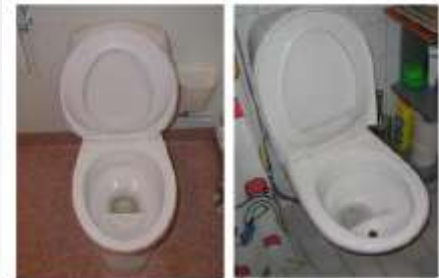
Figure 8. Two urine-diverting toilet models on the Swedish market. a) Gustavsberg Nordic 393U and b) WM-Ekologen DS.
